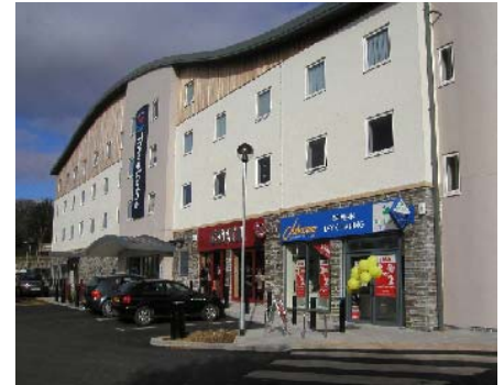
St. Austell Travelodge, Costa Coffee and Johnsons trading (February 2006).
